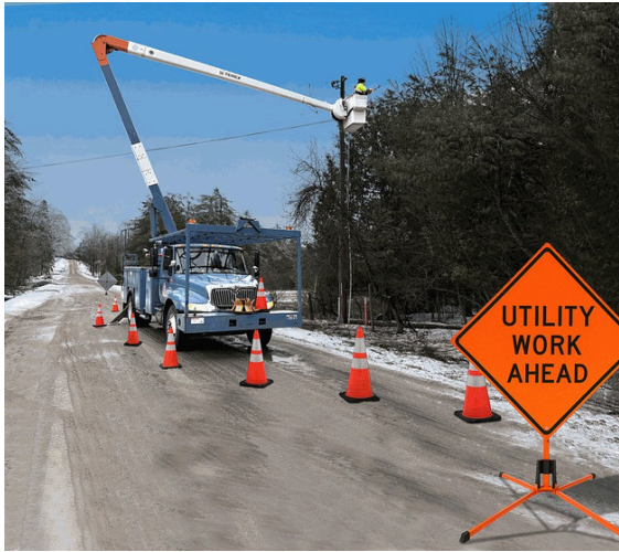
Figure 3-4 – Utility Work Ahead sign
